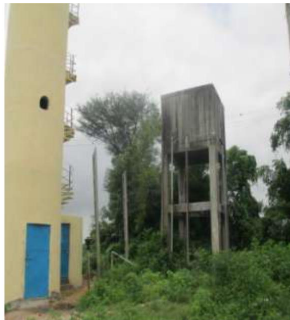
FIGURE 4.4.1 ELEVATED STORAGE TANKS (1 LAKH LITERS)
