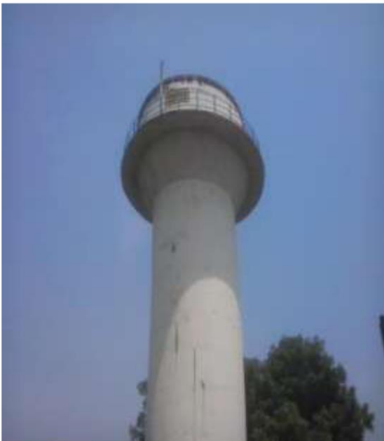
FIGURE 4.4.1 ELEVATED STORAGE TANKS (1 LAKH LITERS)
